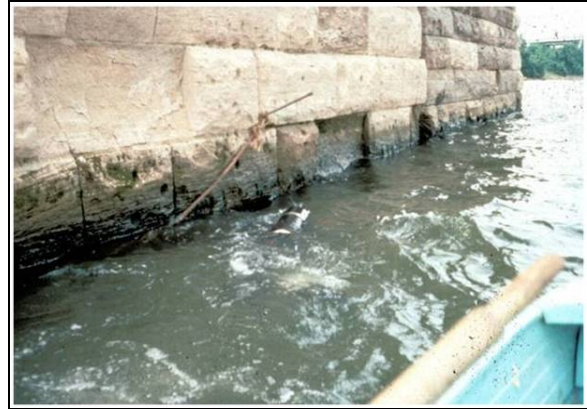
Figure 3-3 Deteriorated Masonry
