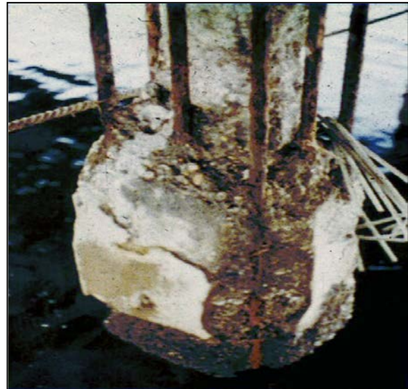
Figure 3-10 Concrete Pile During Repair
