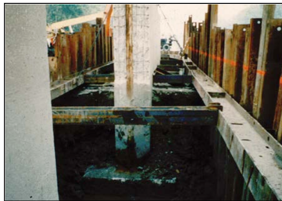
Figure 5-7 Cofferdam Used for Pier and Foundation Extension
