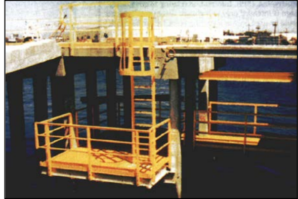
Figure 4-10 Platform Built of Fiber Reinforced Plastic Members and Decking
