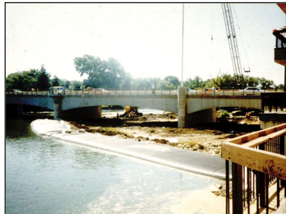
Figure 5-9 Water Filled Tubular Barrier
