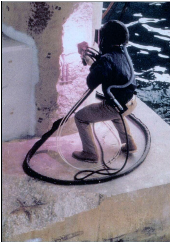
Figure 9-8 Application of Sprayed Zinc
