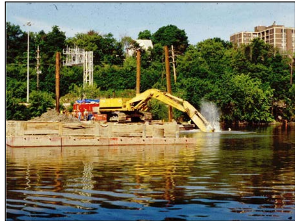
Figure 6-14 Hydraulic Excavator Performing Underwater Excavation
