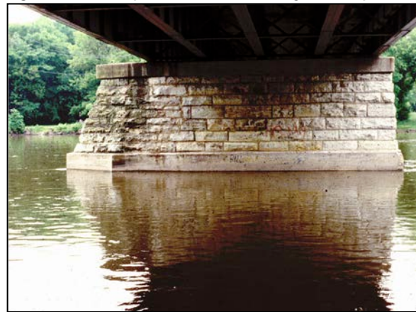
Figure 7-8 Concrete Encasement of Stone Pier
