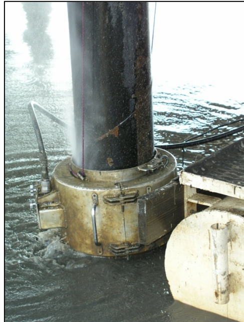
Figure 6-16 Contractor Built Pile Cleaning System (Photo appears courtesy of Substructure, Inc.)
