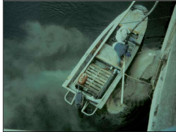
Figure 5-4 Grout Discharge into River
