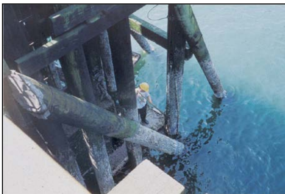
Figure 8-8 Pile Cleaning
