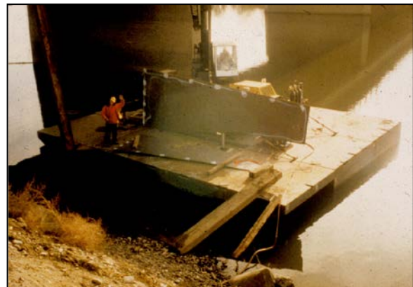
Figure 7-11 Steel Plate Form Trimmed to Fit Stream Bed
