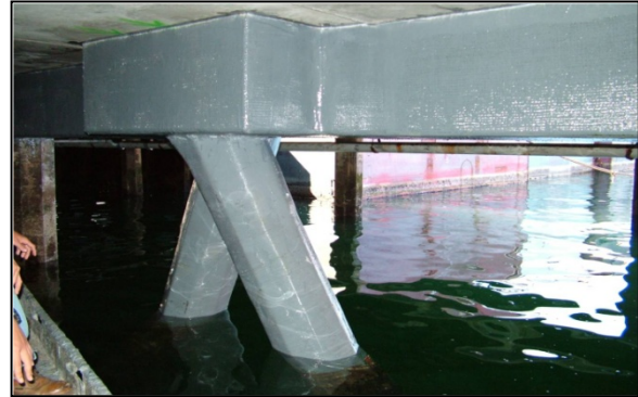
Figure 8-29 FRP Strengthening of Concrete Piles and Pile Cap
