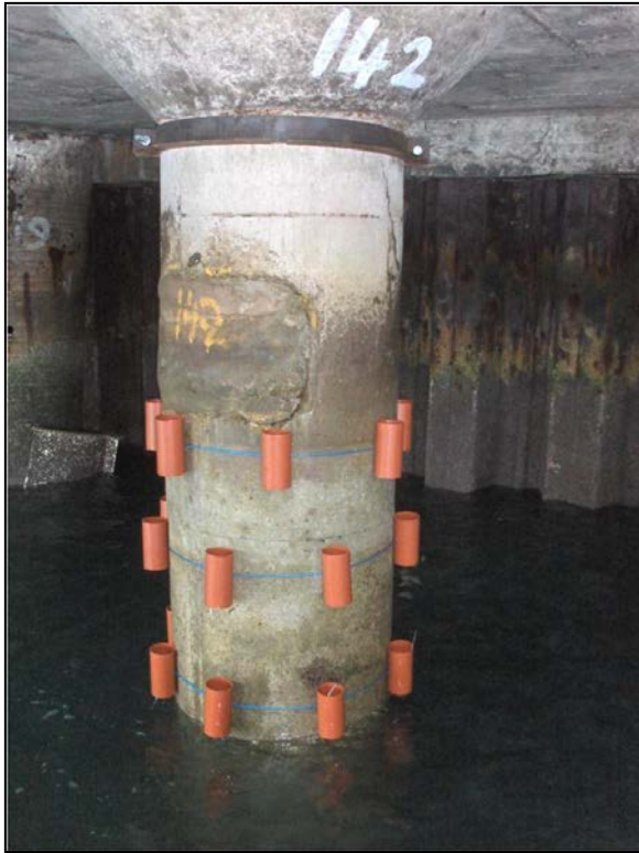
Figure 8-15 Formwork Spacers in Place
