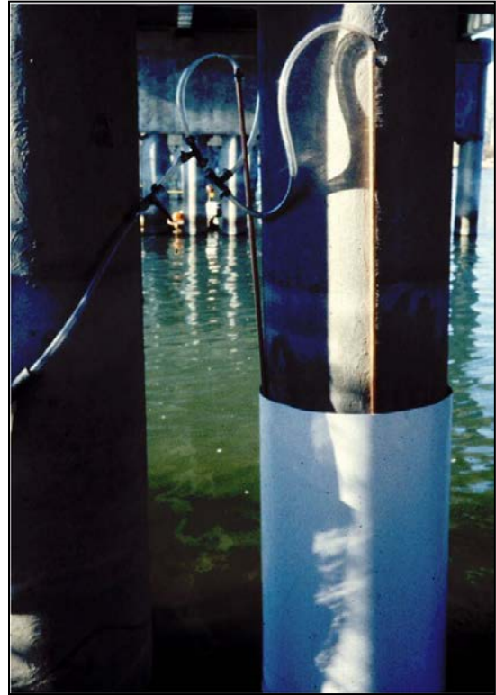
Figure 8-24 Epoxy Placement Pipes in Form
