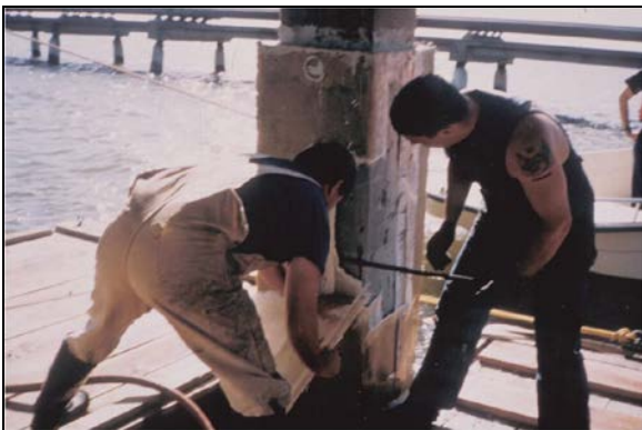
Figure 8-27 Removal of Pile Jacket to Verify Installation Procedures
