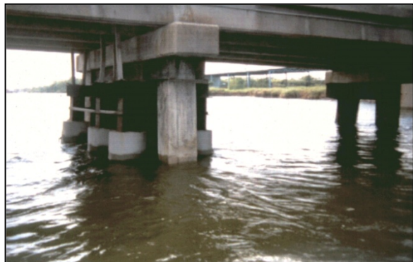
Figure 8-4 Supplemental Pile Bents (Crutch Bent)
