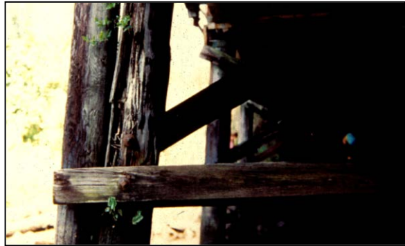
Figure 8-2 New Pile Driven Outside of Damaged Pile
