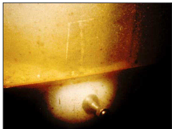
Figure 7-2 Permanent Steel Plate Form Secured with Expansion Anchor
