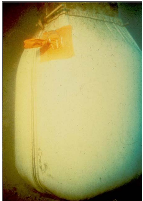
Figure 8-20 Completed Underwater Fabric Form Repair
