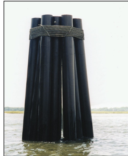
Figure 4-7 Polymer Pile Dolphin
