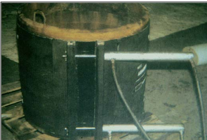
Figure 8-12 Cutaway of Wraps with an Interim Protective Layer. The Wrap Uses a Proprietary Clamp Closure System
