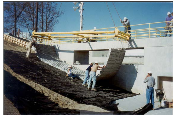
Figure 7-15 Articulated Concrete Block System Being Installed
