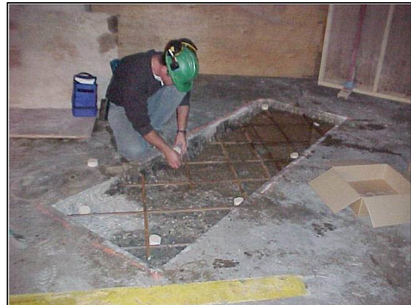
Figure 9-10 Galvanic Sacrificial Embedded Anodes Along Edge of Repair
