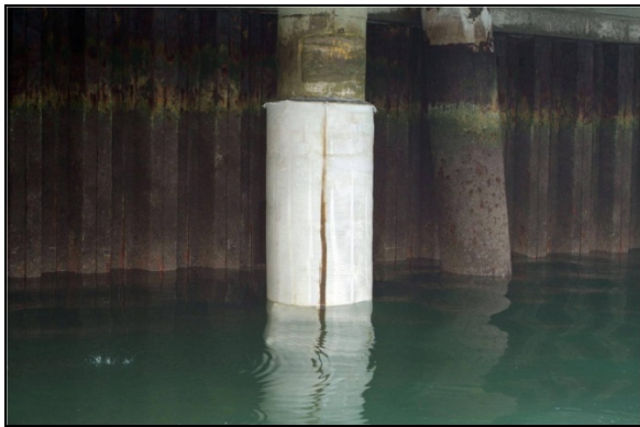
Figure 8-19 Completed Fabric Form Jacket
