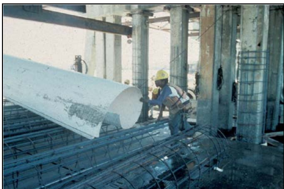
Figure 8-21 Semi-rigid Stay-in-Place Form; Note Also the Reinforcing Cages Sit Awaiting Forms
