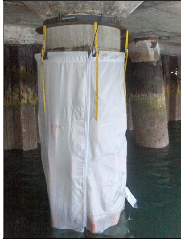
Figure 8-16 Fabric Form Installation
