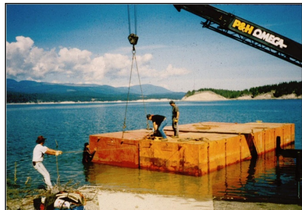
Figure 6-4 Sectional Barges Being Assembled
