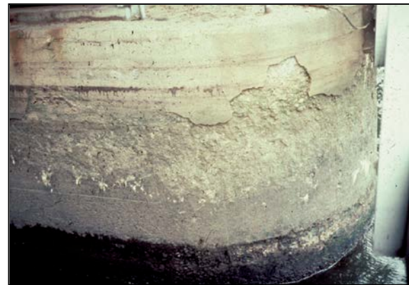
Figure 3-5 Deteriorated Concrete
