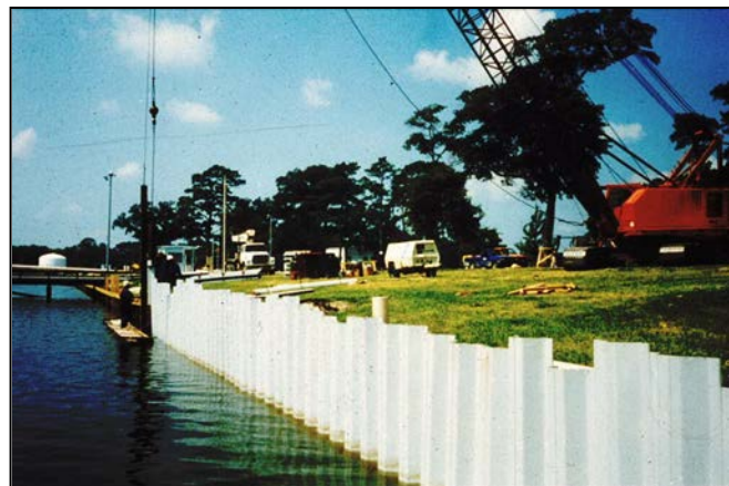
Figure 4-9 Polymer Sheet Pile Wall
