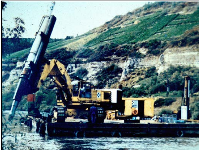
Figure 6-15 Specialized Underwater Hydraulic Hammer
