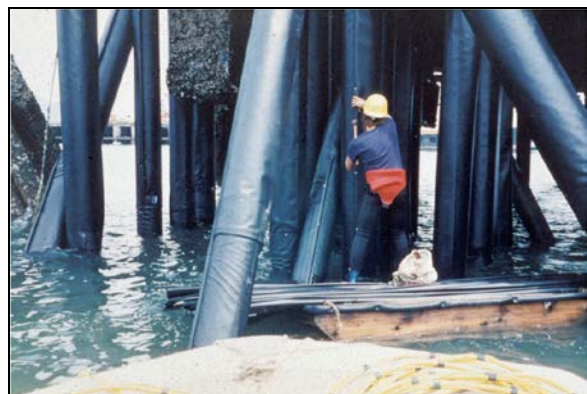
Figure 8-9 Pile Wrap Installation
